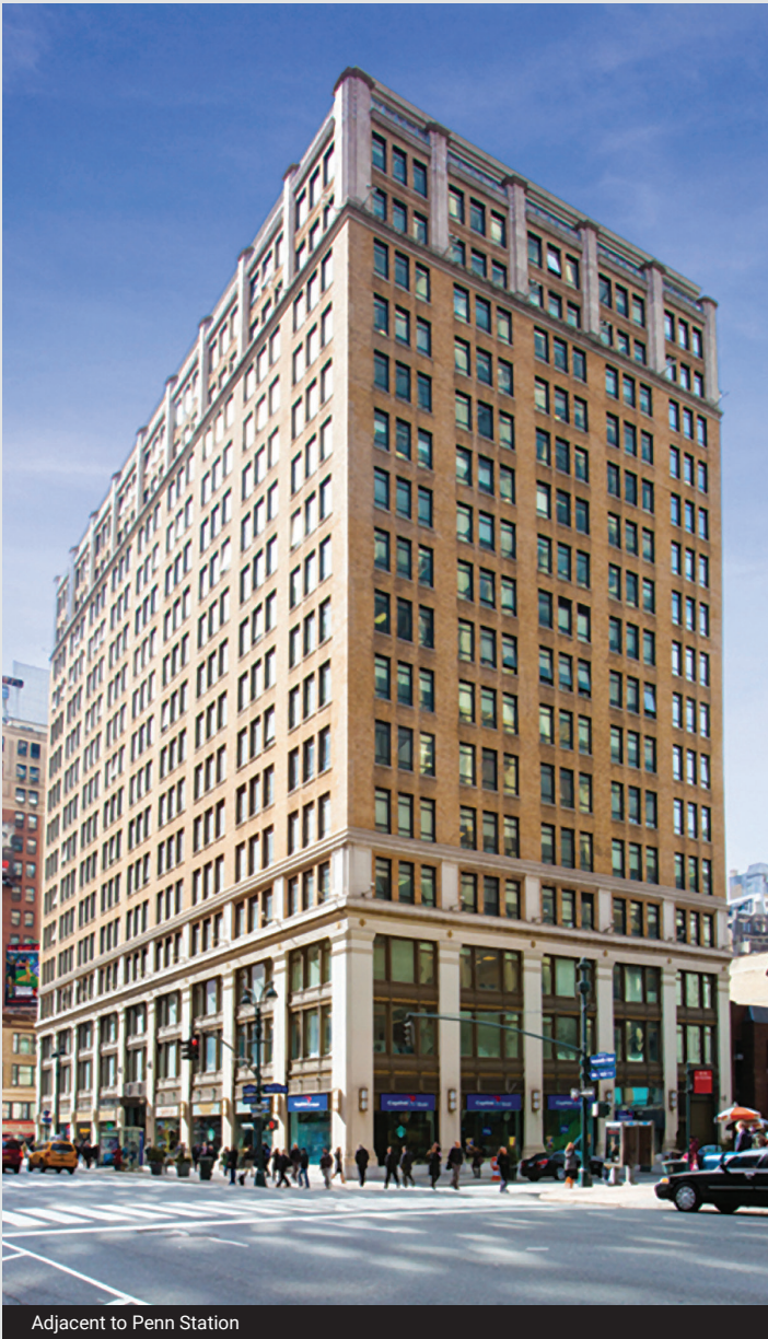
Adjacent to Penn Station
