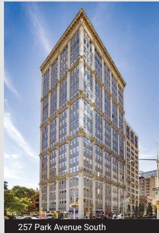
257 Park Avenue South
